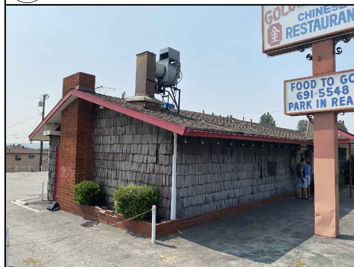
4 EXISTING BUILDING (EAST SIDE)
