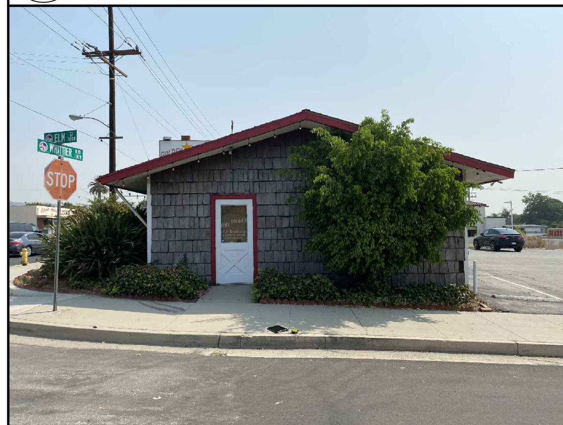
3 EXISTING BUILDING (WEST SIDE)
