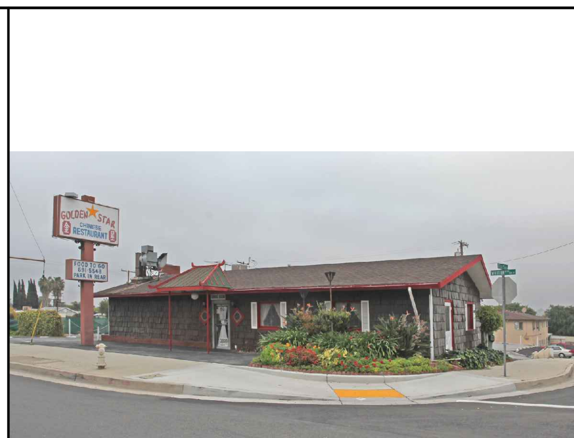
1 EXISTING BUILDING (NORTH SIDE)
